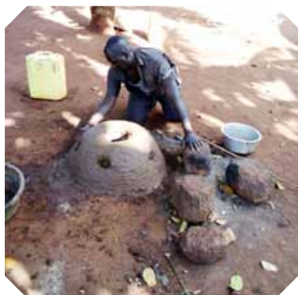
Transition from 3 fire stone to stationed energy saving cookstove
